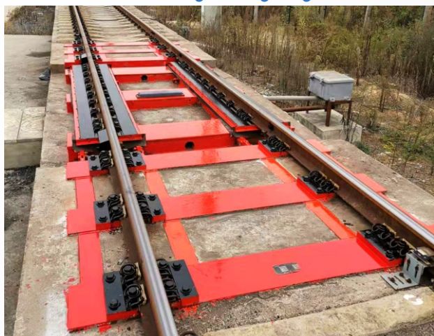
Shallow foundation pit concrete foundation form
