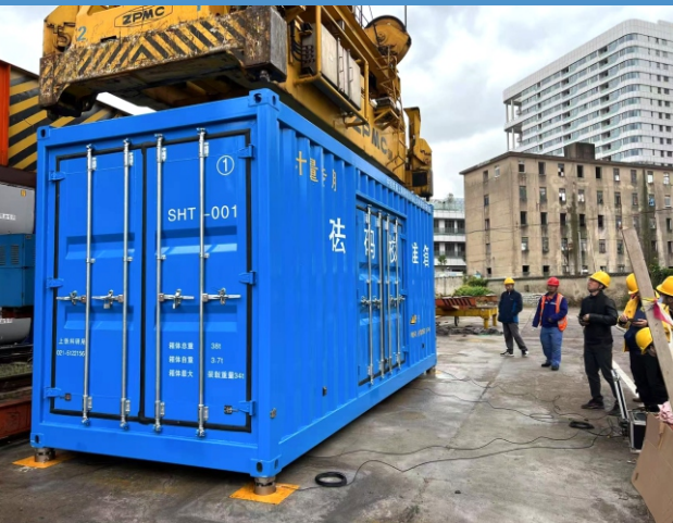
Weight box used on site at Shanghai Beijiao Freight Yard
