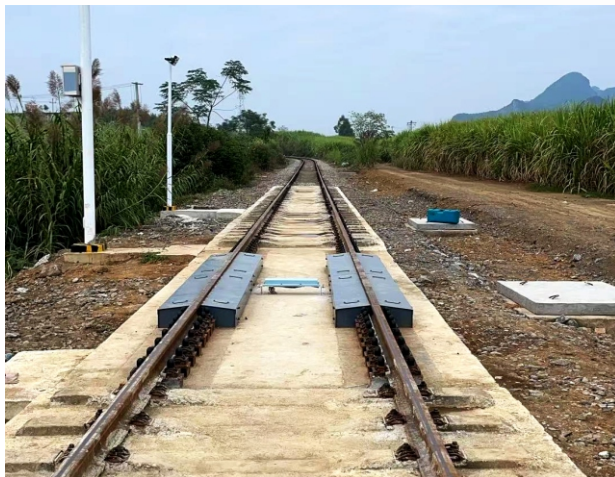
Foundation form with pre-embedded steel plates without foundation pit
