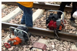
Sensor hole machining
