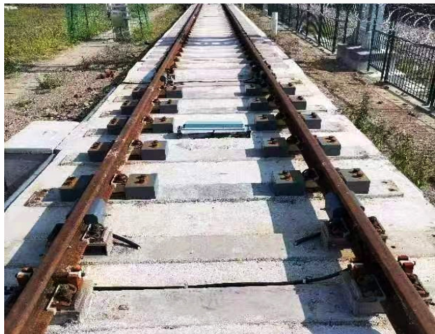
Foundation form with special sleepers without foundation pit
